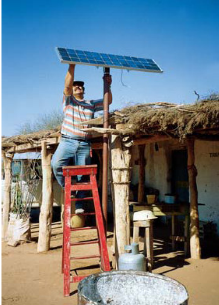
Source: Fraunhofer ISE. Solar home system in Argentina
